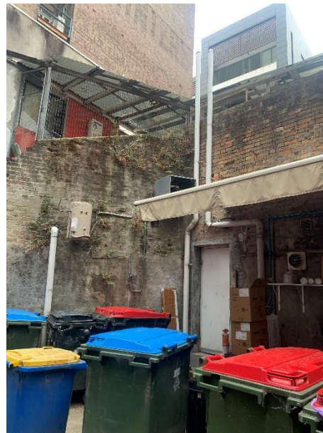
Figure 22 – Rear dock/service yard accessible via Foster Lane.
