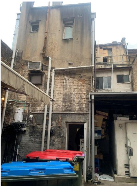
Figure 21 – Rear dock/service yard accessible via Foster Lane.
